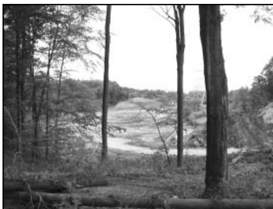
Red Hill Valley under construction. Photo courtesy of Lake Ontario Waterkeeper.
