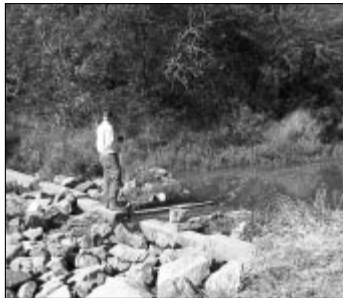
Canborough weir pre-remediation. Photo by Dan Mcdonell.
