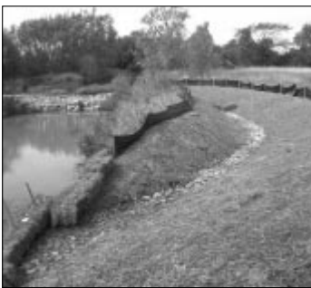
Canborough weir during remediation. Photo by Dan Mcdonell.
