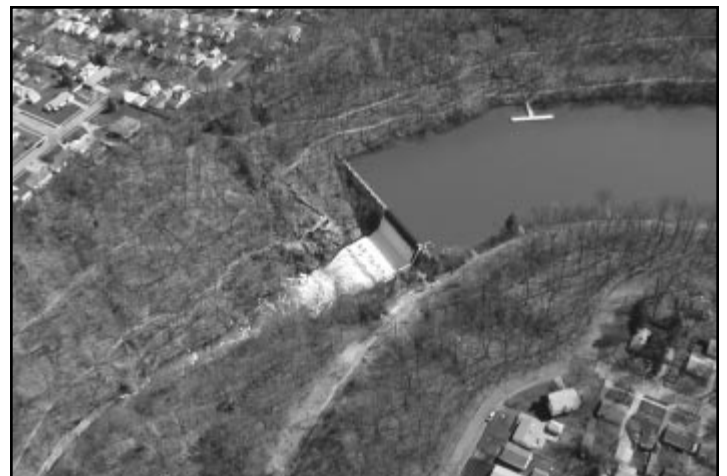
Gorge Metro Park is a 140 acre natural preserve in the urban core of Akron and Cuyahoga Falls. The proposed hydro project will require building roads, parking lots, a power house, transmission lines, concrete supports and a plume. This construction will cause erosion on steep slopes, loss of natural habitat in the urban core and water quality degradation. Photo courtesy of Friends of the Crooked River.
