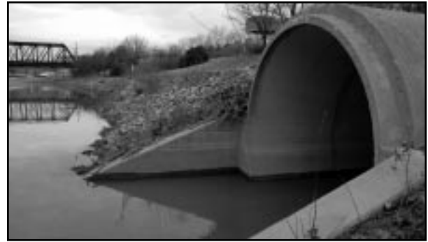
Any moderate to heavy rain storms lead to the dumping of untreated sewage into our waterways from pipes like this one on Ohio's Scioto River.
