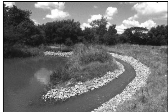
Fish barrier remediation with by-pass channel, photo courtesy of NRC.
