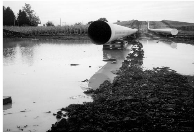
“The Guardian Pipeline construction.”
