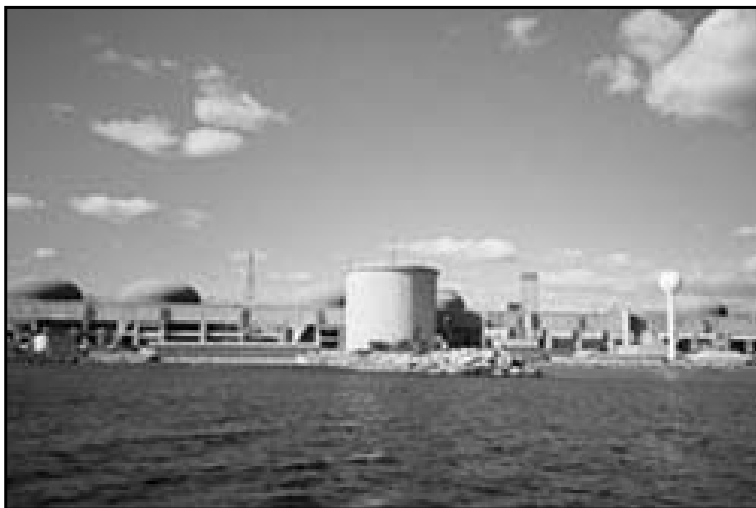
Pickering Nuclear Generating Station on Lake Ontario. Photo courtesy of Lake Ontario Waterkeeper.
